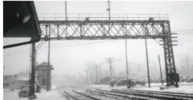
A souvenir from one of the author's visits to Athens. Shot with a Kodak box camera in the late 1940s, this view captures the tower, left, and the signal bridge controlling the approach to Sayre Yard. The shot is from the Athens station platform. David Marcham
