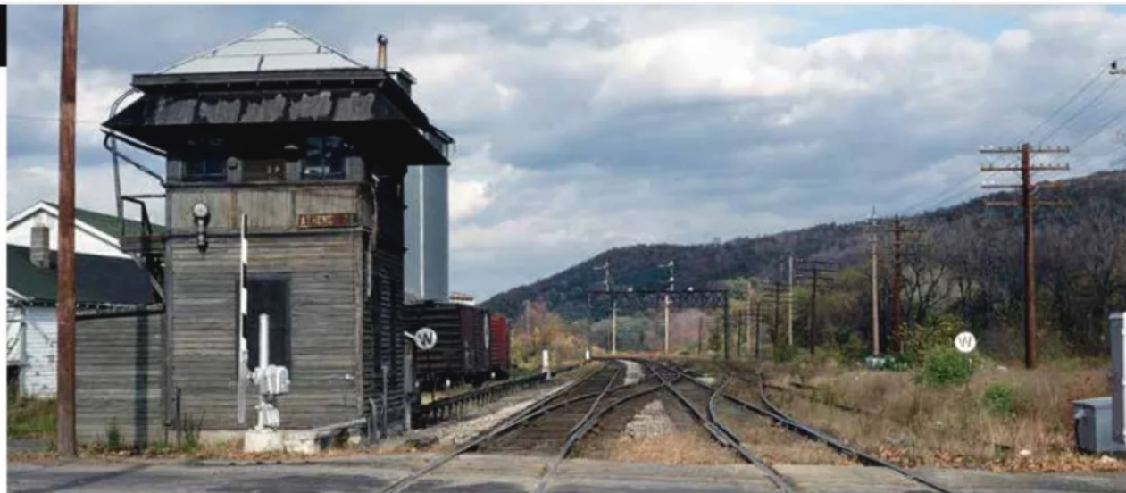
This view is looking railroad west at Athens Tower. Along the track at left is the equipment connecting the tower to the signal bridge. Main Street is in the foreground. Robert Archer
