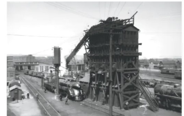
One of the railroad's passenger-hauling Pacifics takes on coal from the facility at Sayre. These 4-6-2s were typically on the point of LV's premier passenger train, the Black Diamond . David Marcham
