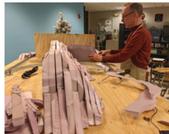
To build our mountain, we stacked layers of foam on end. Here, David is fitting a section near the tunnel, using a scrap piece of plywood as a stand-in for the building flats, shown on the previous page.
