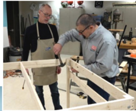
David Popp (left) and Hal Miller made the frame from standard 1 x 4 and 2 x 2 lumber with a 3/4" plywood top. We designed our train table (shown below) to be sturdy yet easy to assemble.
